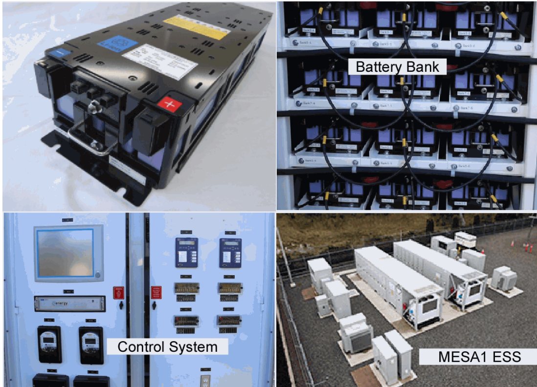
Figure 1.2. MESA-1a Module, String, Control System, and MESA-1 Site with all Major Components
