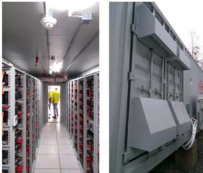
Figure 1.9. Thermostats inside the Container (left) Control Ductless Heat Pump/Air Conditioning Units (right)
