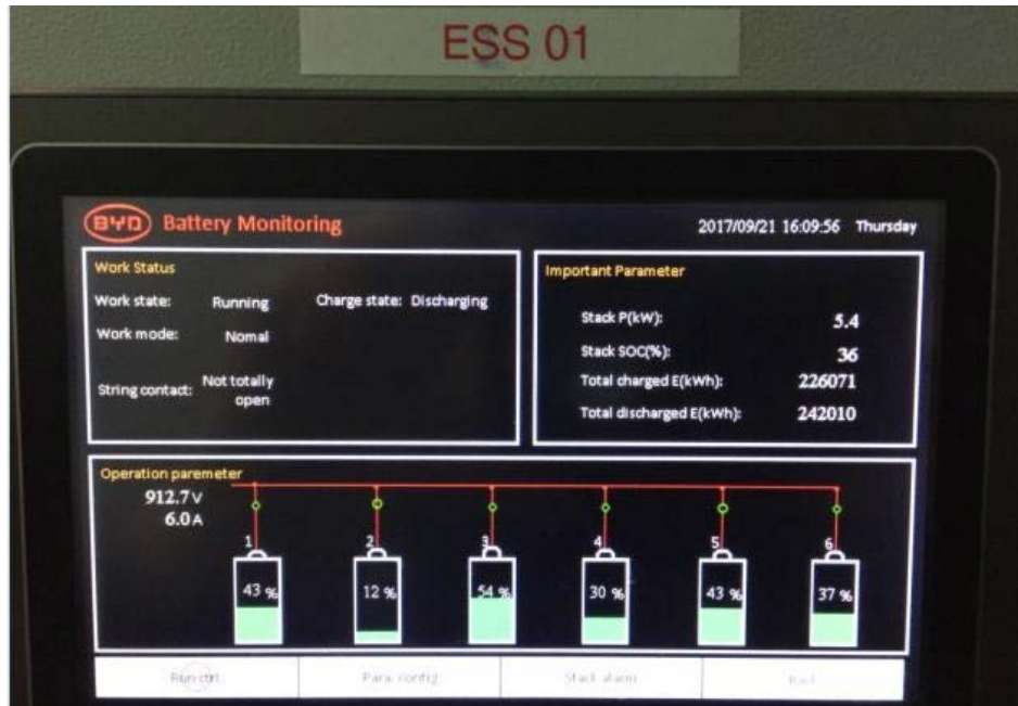
Figure 1.4. BYD String Status for Container 1
